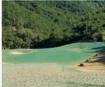
Golf Course Construction
